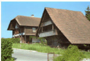
2.11 Speicher, Räzlrain 6 a
