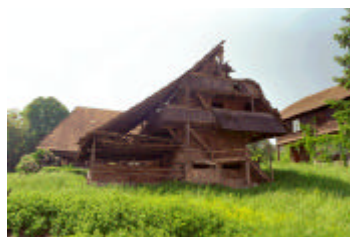
2.11 Speicher, Räzlrain 6 a
